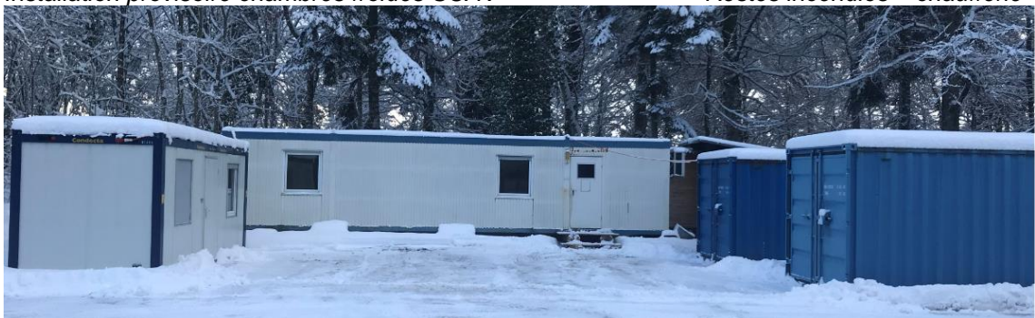
Installation provisoire centre forestier
