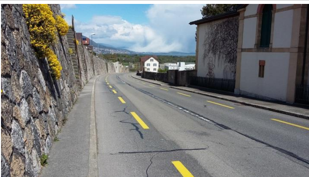
Route cantonale 1002, Cortailod
