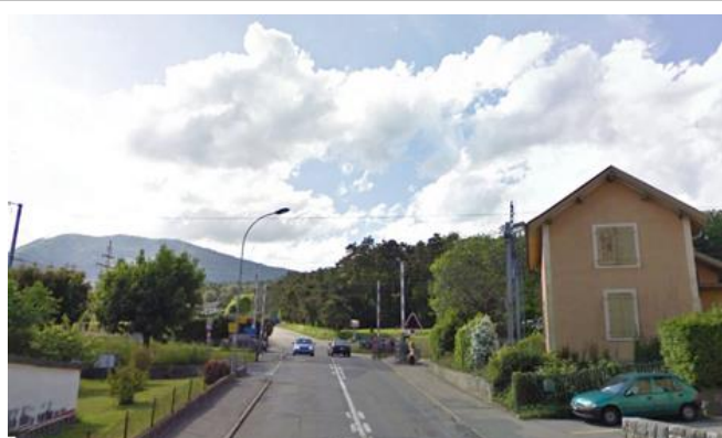
Route cantonale 173, Rochefort
