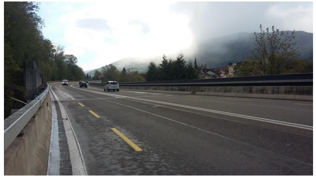
Route cantonale 5, Boudry
