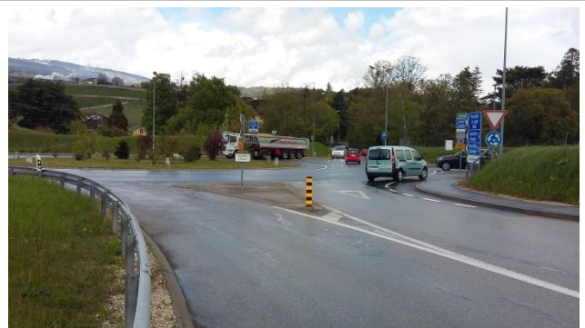
Route cantonale 1002, Boudry
